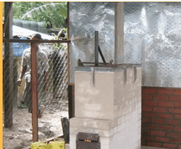
Small-scale incinerator for treatment and disposal of waste, minimizing emissions, and reducing occupational exposures and other hazards in line with best practice principles.
