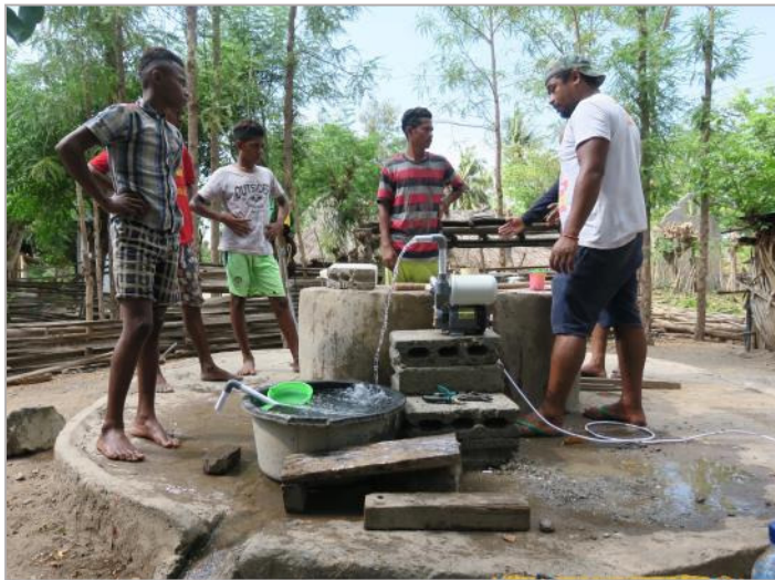
Installing a new pump to aid in irrigating vegetable gardens.
