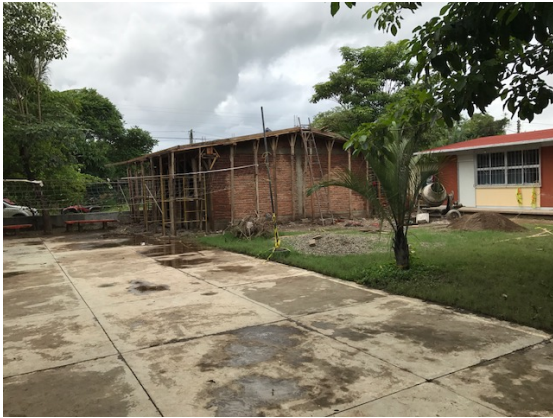
Las Palmas secondary – new classroom
