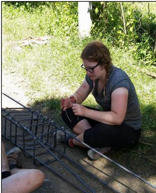
Making of the beams... my new found skills!
