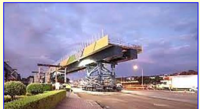
A section of bridgework for the Darlington Upgrade Project constructed off site ready for transport into position.
