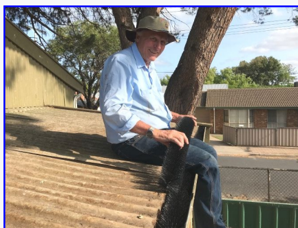
PP Malcolm installing the new gutter guard on our shed roof
